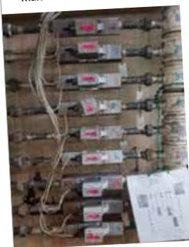
9 secondary small pipes with water meters. These meters were installed to make sure a stable flow rate. If the flow rate goes down, it would cause a problem of the induction hardening machine. Therefore, the pipes had to be cleaned manually every 2-3 months.
